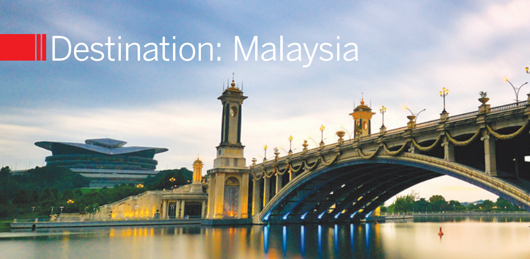
A modern bridge leading to the Putrajaya International Convention Centre
