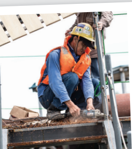
Technicians carefully securing each portion of the backdrop.
