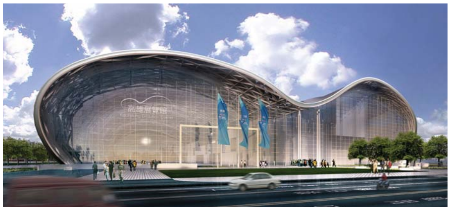
The new Kaohsiung Exhibition Center gives the city ammunition to court large events
