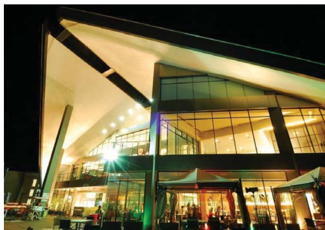
(From top) Aerial view of the sprawling Grand Kawanua International City and Novotel Manado Golf Resort & Convention Center
